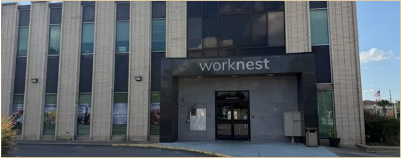
Main entry · Ohio Avenue South
